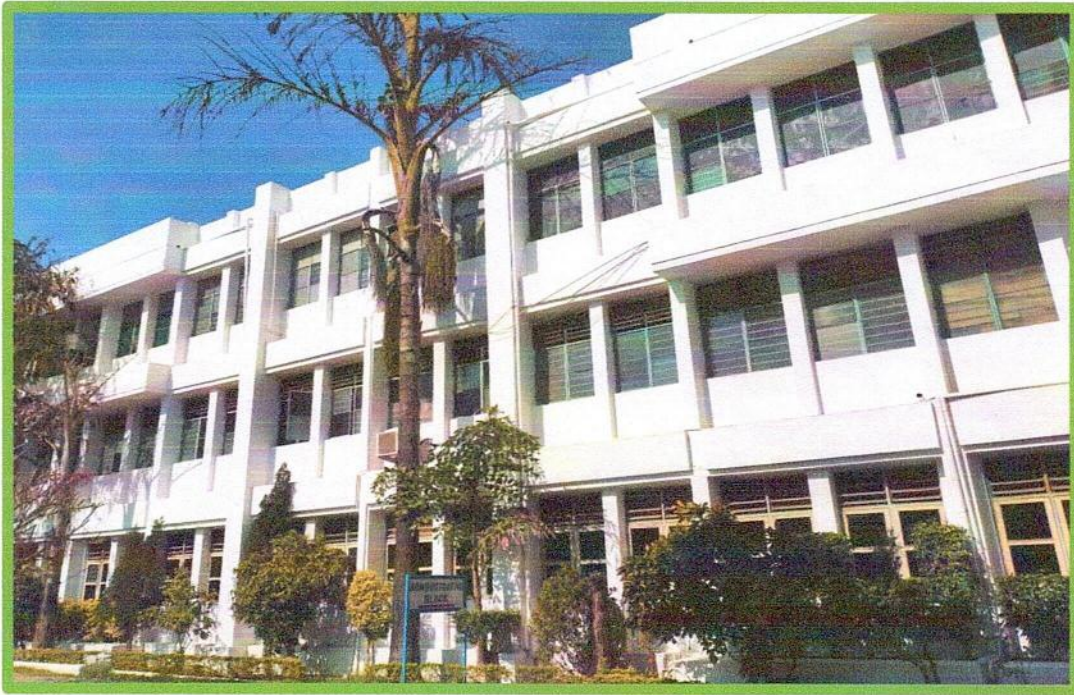
Figure4: Large windows provided for natural ventilation reducing power consumption
